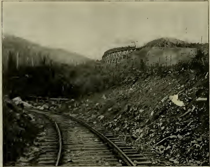
CROWN TRESTLE NEAR ROSSLAND, B. C.
